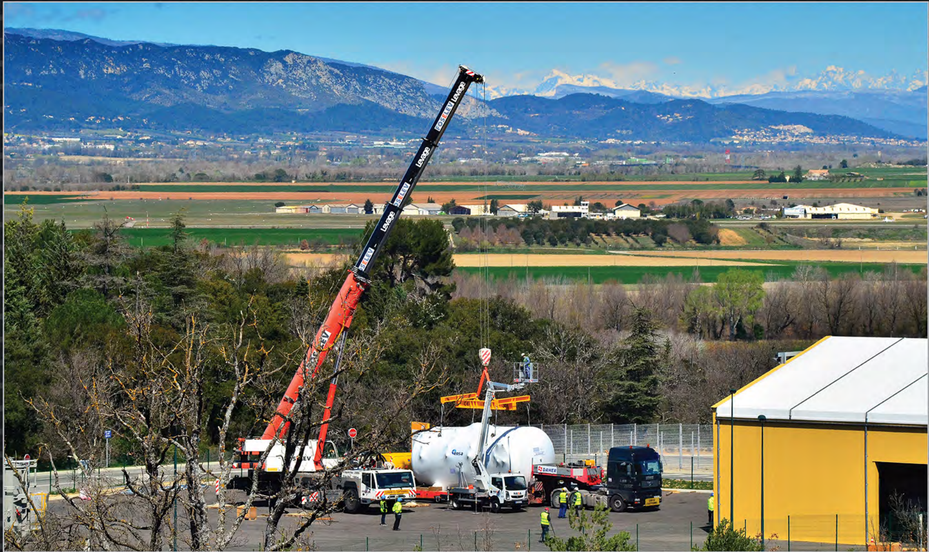
Five on-site warehouses are now in place for the storage of in-kind contributions to ITER. (Pictured: a water detritiation tank procured by Europe.)
