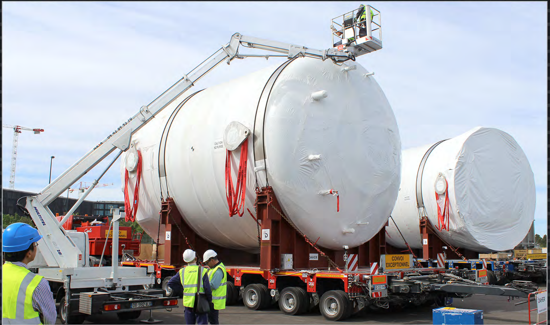
The first drain tanks for the tokamak cooling water system were delivered to the ITER site in May and the remainder of the tanks arrived at the site in September 2015.
