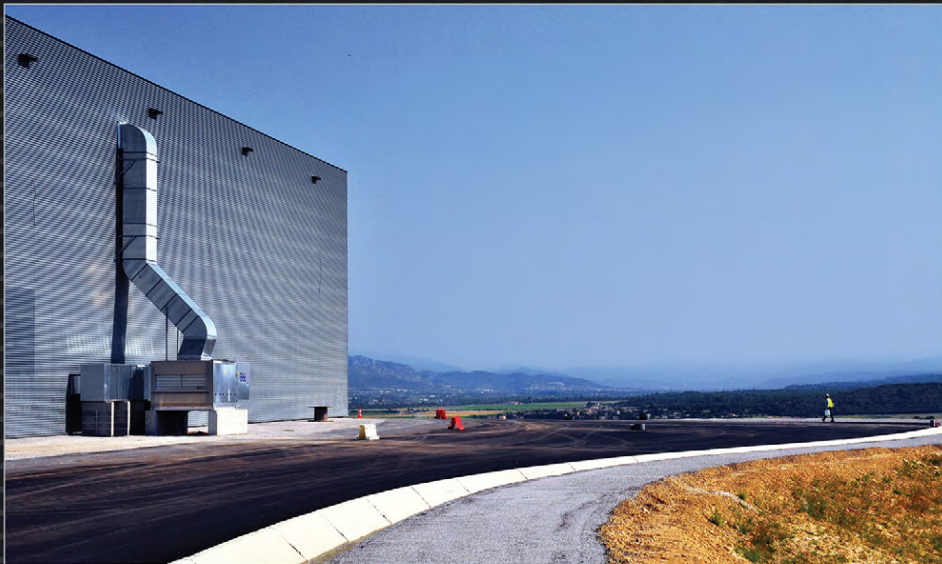
This 9,000 m 2 storage facility was erected in 2015 by the ITER Organization to house machine and plant components sent by the ITER Domestic Agencies. It is the largest of four warehouses on site.
