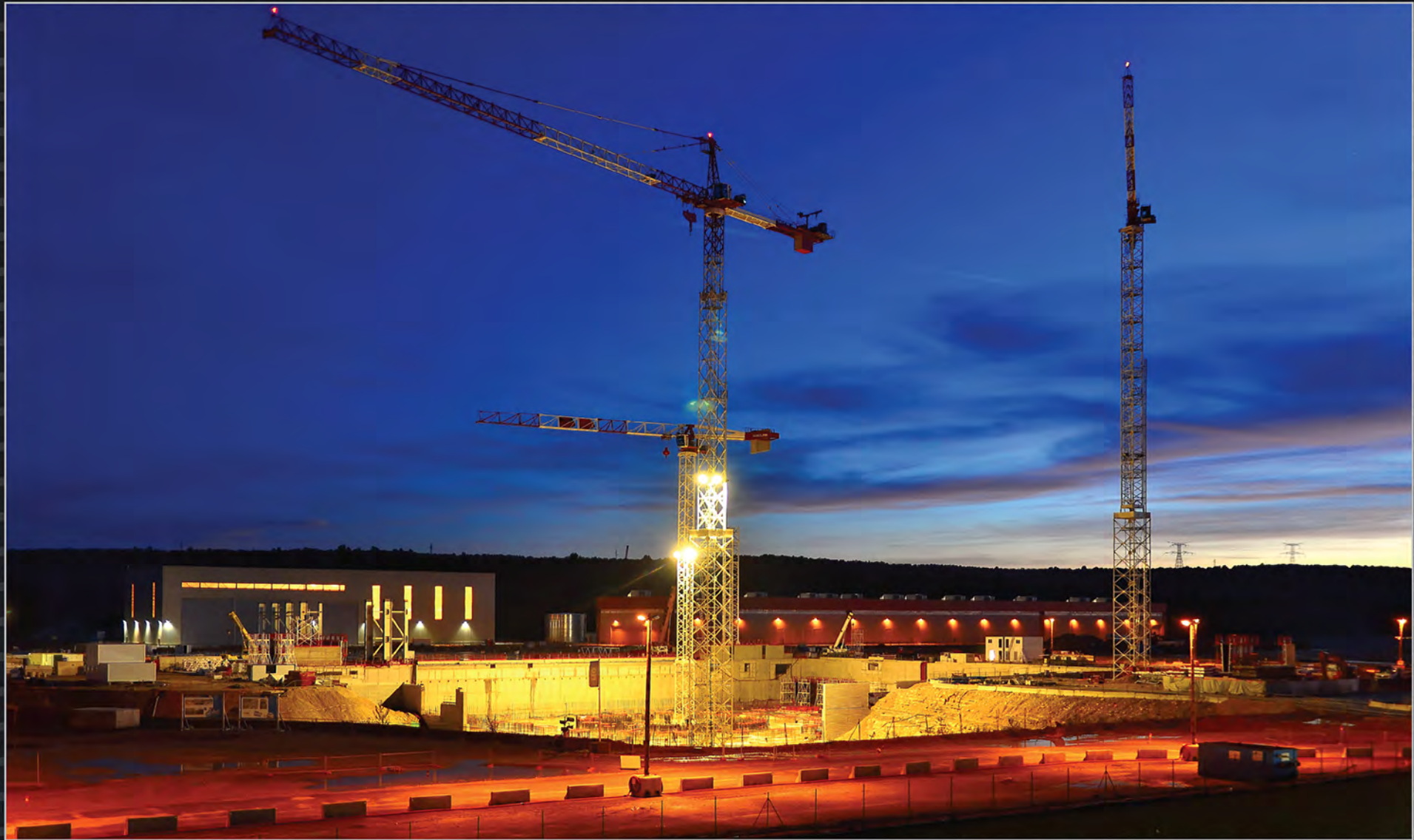
The end of a work day on the ITER site. November 2014
