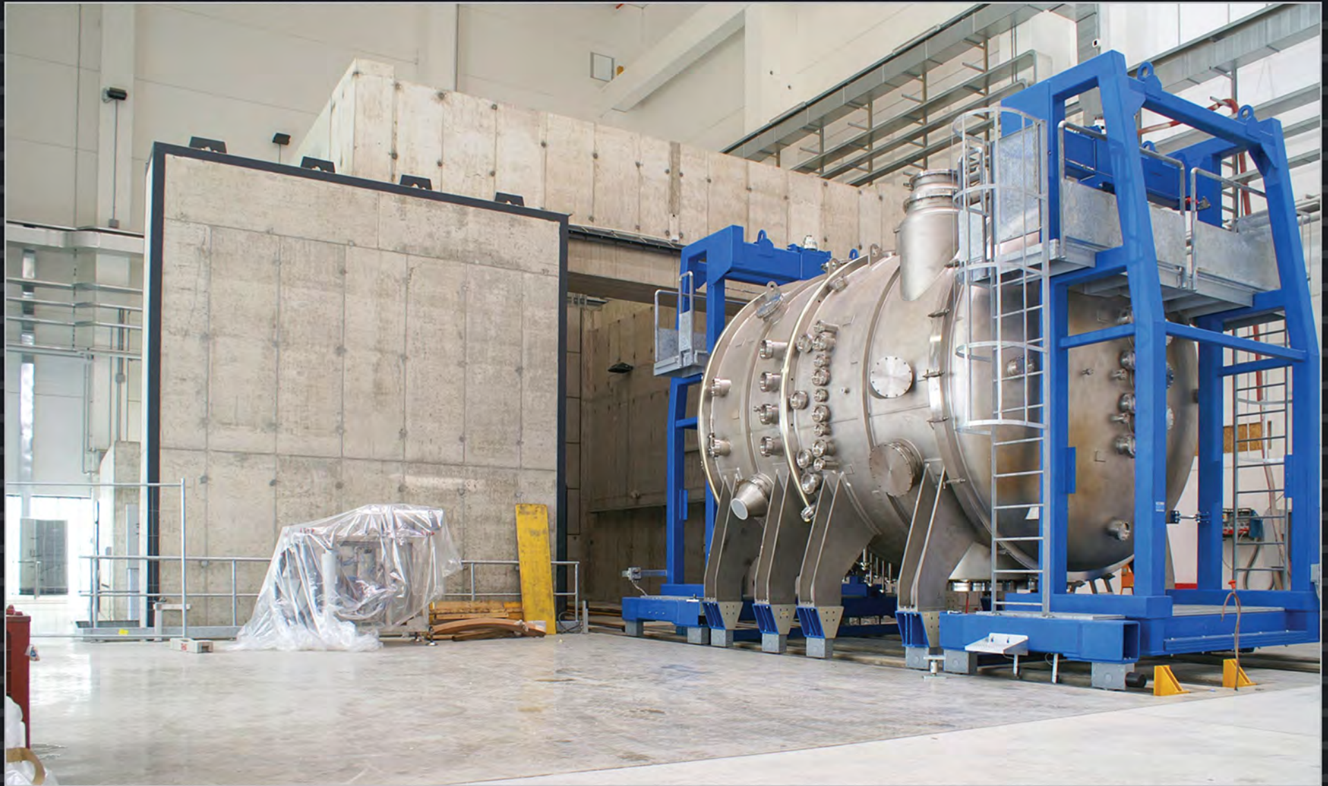
At the PRIMA facility in Padua, Italy, ITER neutral beam technology will be tested in advance of operation on SPIDER (an ITER-scale radio-frequency negative ion source) and MITICA (a full-scale ITER neutral beam injector at full acceleration voltage and power). Europe, Japan and India are all contributing components. In 2015, Europe delivered the SPIDER vacuum vessel pictured above.
