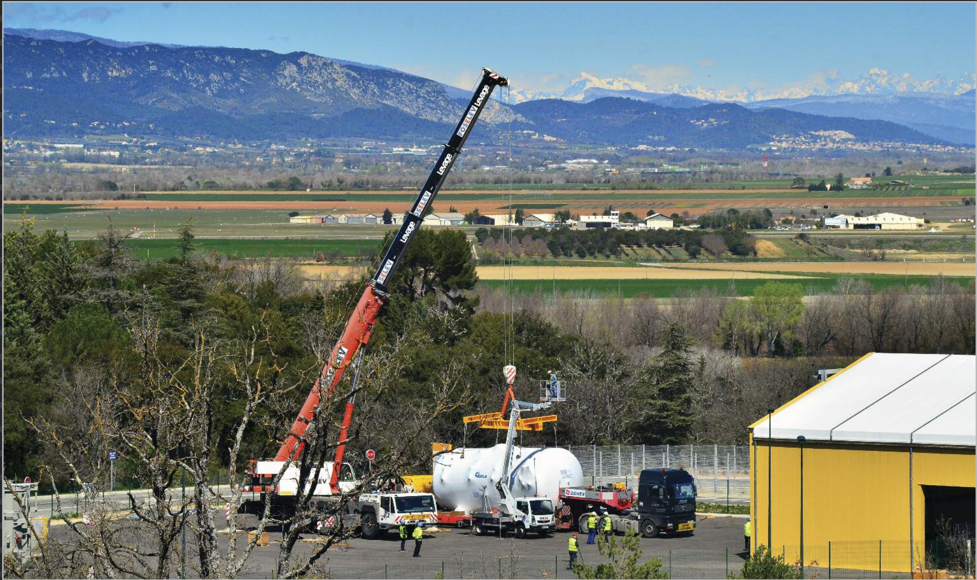
Five on-site warehouses are now in place for the storage of in-kind contributions to ITER. (Pictured: a water detritiation tank procured by Europe.)
