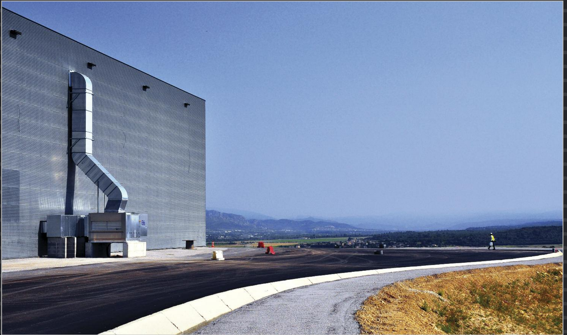
This 9,000 m 2 storage facility was erected in 2015 by the ITER Organization to house machine and plant components sent by the ITER Domestic Agencies. It is the largest of four warehouses on site.
