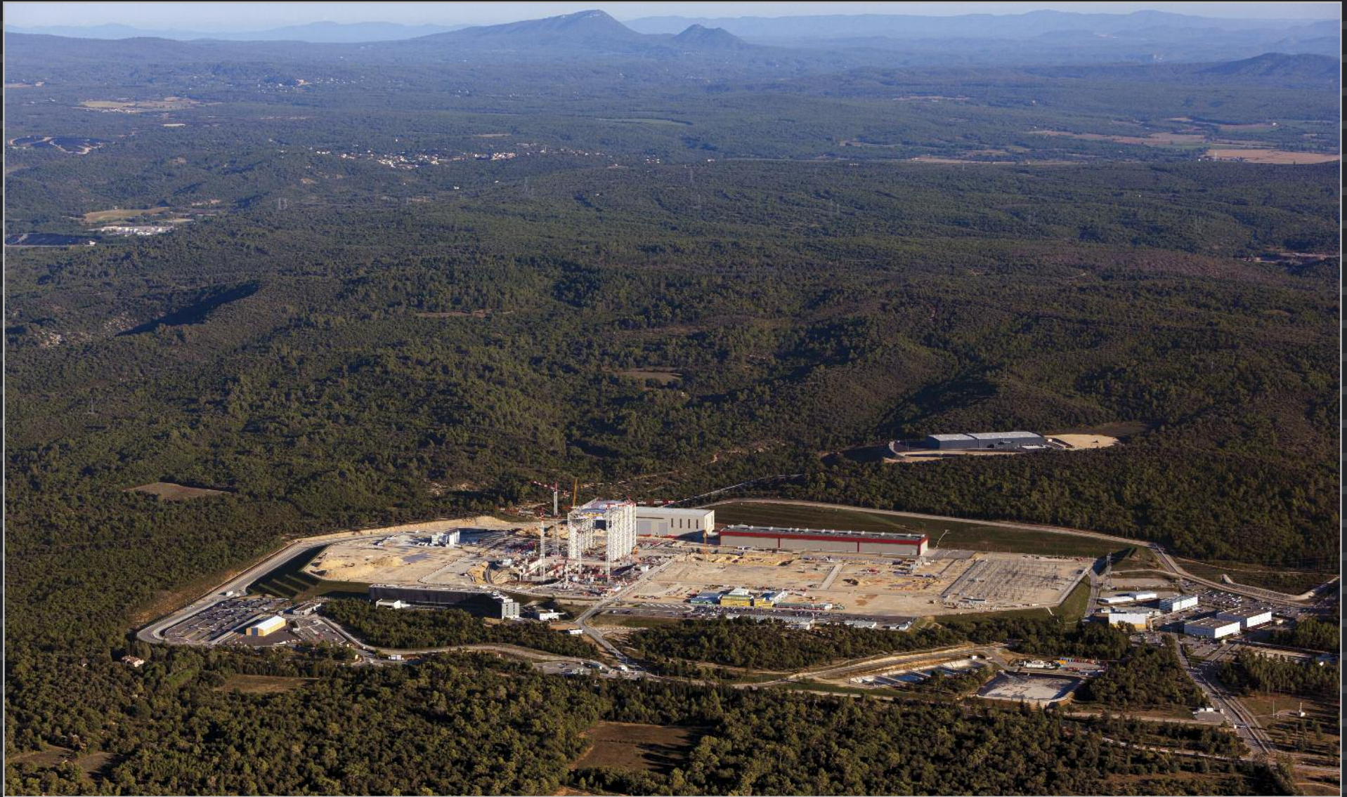
A little over half of the "ITER parcel" has been cleared – the rest remains wooded. Behind the platform, a 9,000 m 2 warehouse is now in place for the storage of delivered components. September 2015
