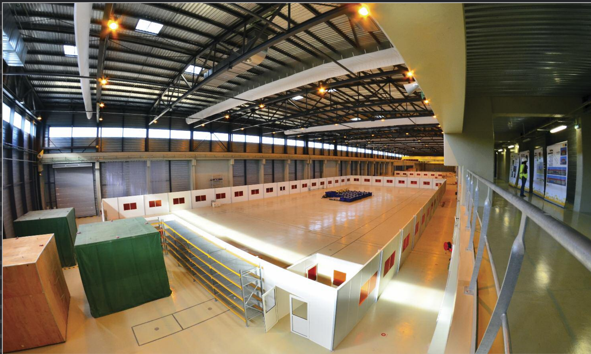
In ITER's largest on-site manufacturing facility, two clean areas are framed out to prepare for the delivery of the first winding tooling. In this 257-metre-long building, Europe will wind and assemble the four largest poloidal field coils. September 2015
