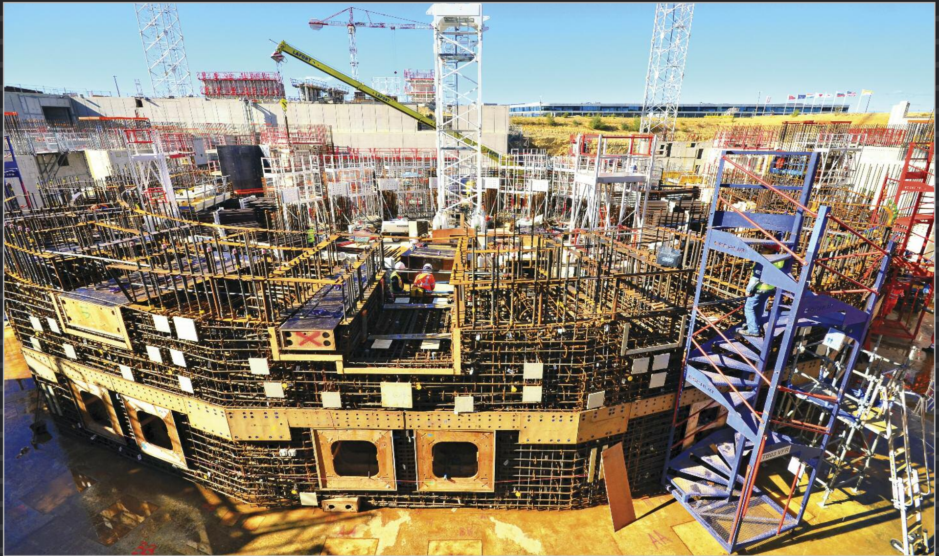
The 3.2-metre-thick ITER bioshield will completely enclose the ITER Tokamak and its cryostat. In the dense reinforcement set into place in advance of concrete pouring, openings are visible for the arrival of electrical and cryogenic supplies.
