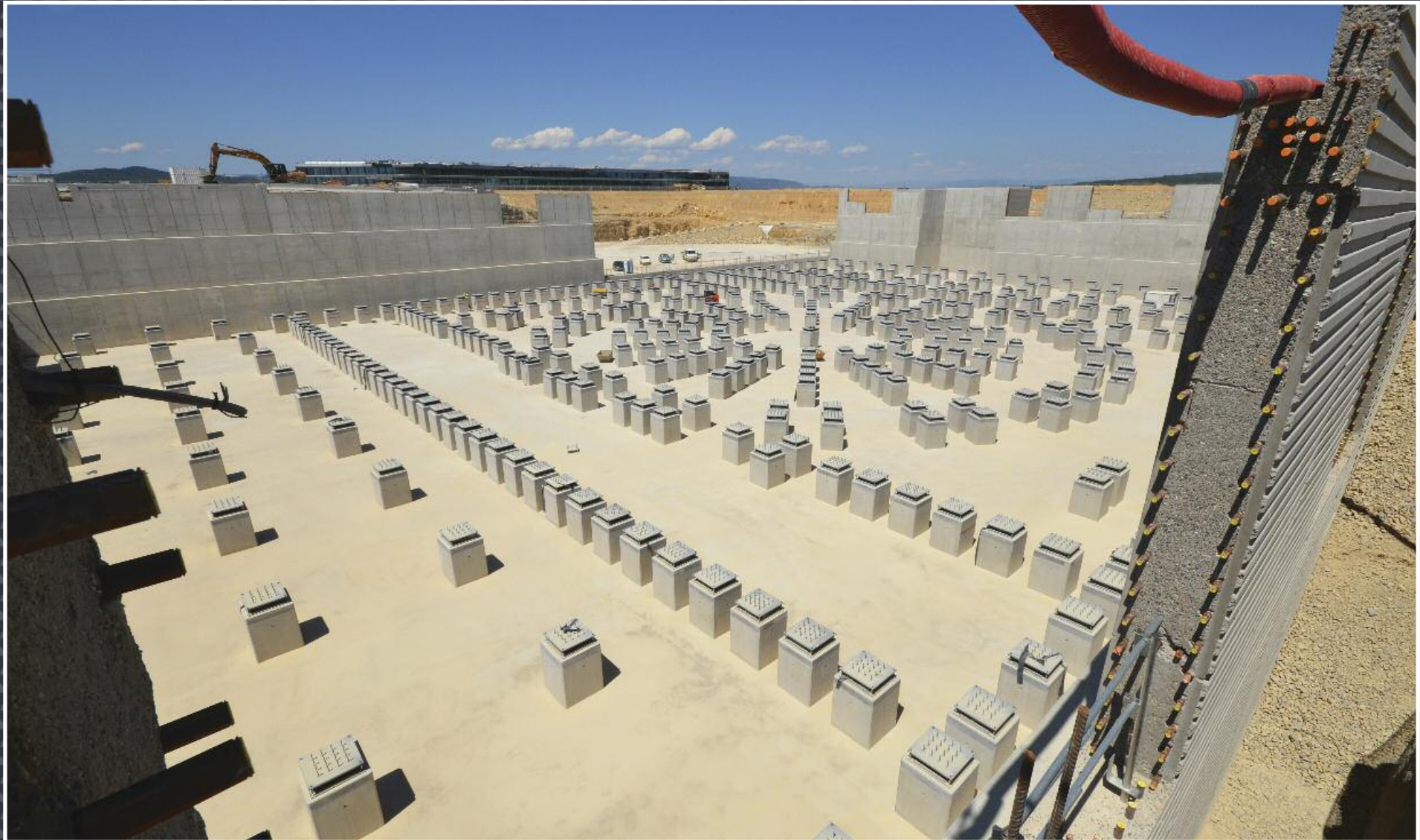
The three buildings of the Tokamak Complex will share a common foundation. In case of a seismic event, 493 steel and rubber seismic pads will absorb ground motion and preserve the integrity and safety of the installation. July 2012
