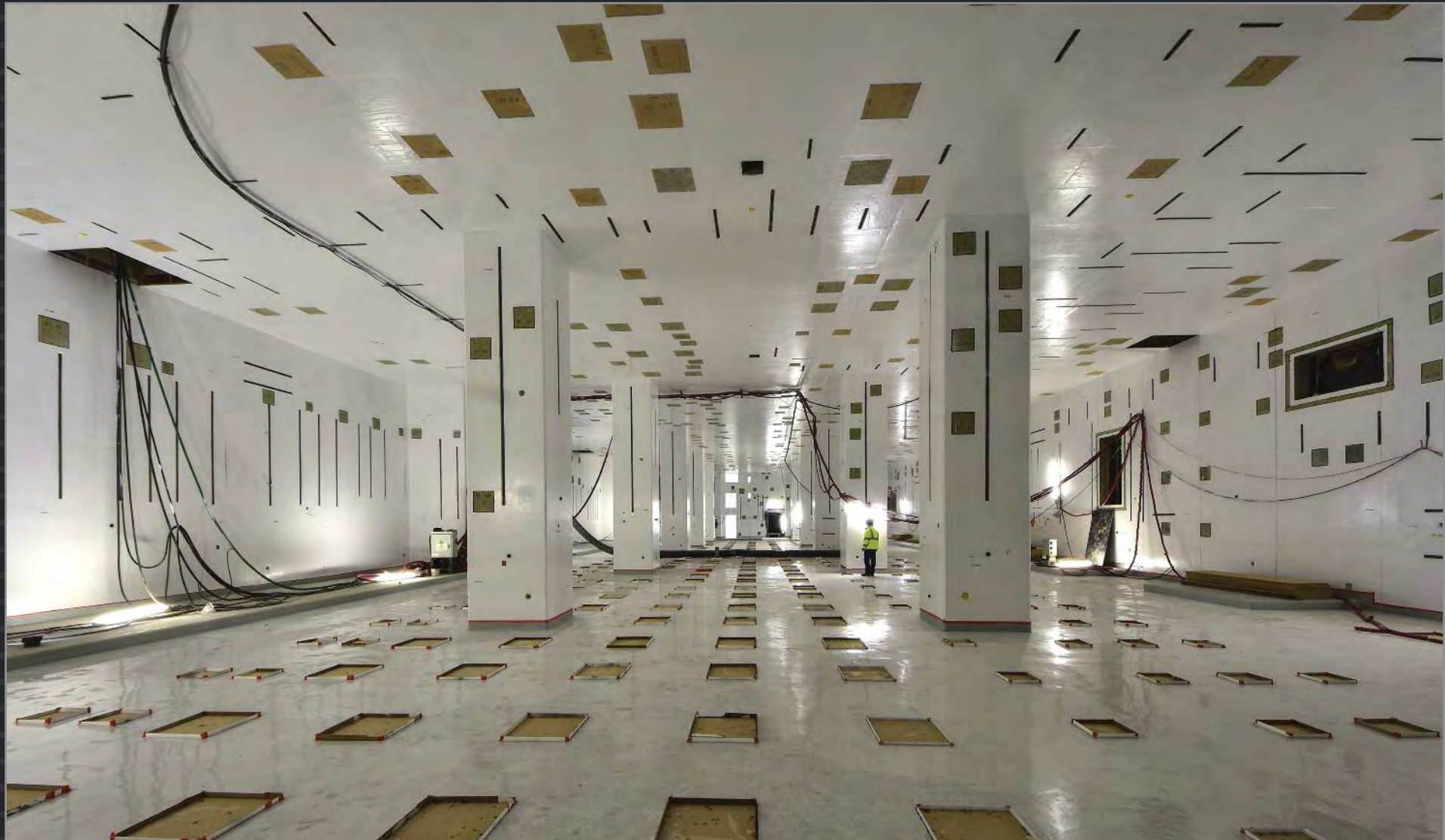
Now painted in white, the lowest basement level of the Diagnostic Building is ready for handover to contractors for systems installation. Embedded plates – for the attachment of system supports – are visible on all surfaces. December 2018
