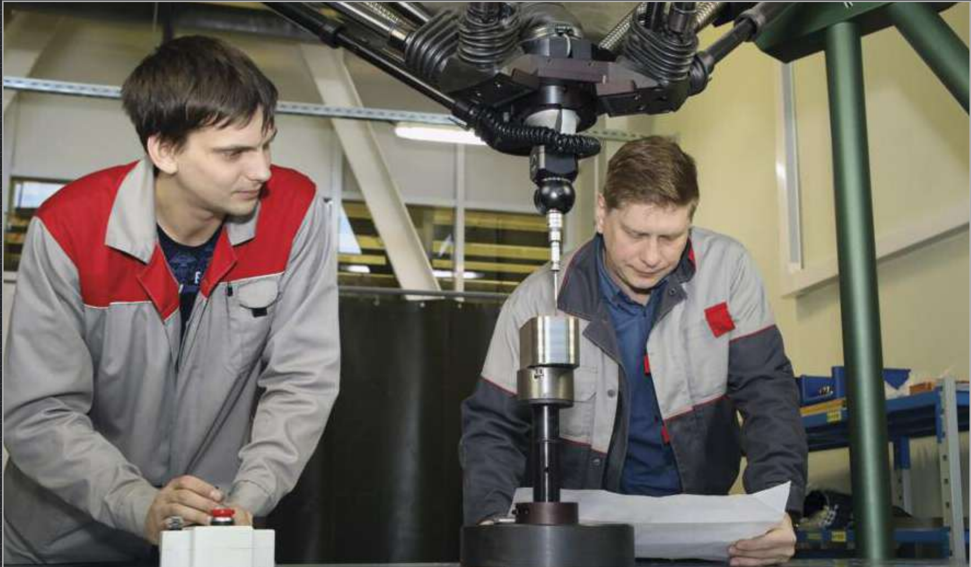
Between the blanket modules and the vacuum vessel, contractors will install low-impedance electrical bridges formed from bimetal "pedestals" (pictured, in testing) and electrical "straps."
