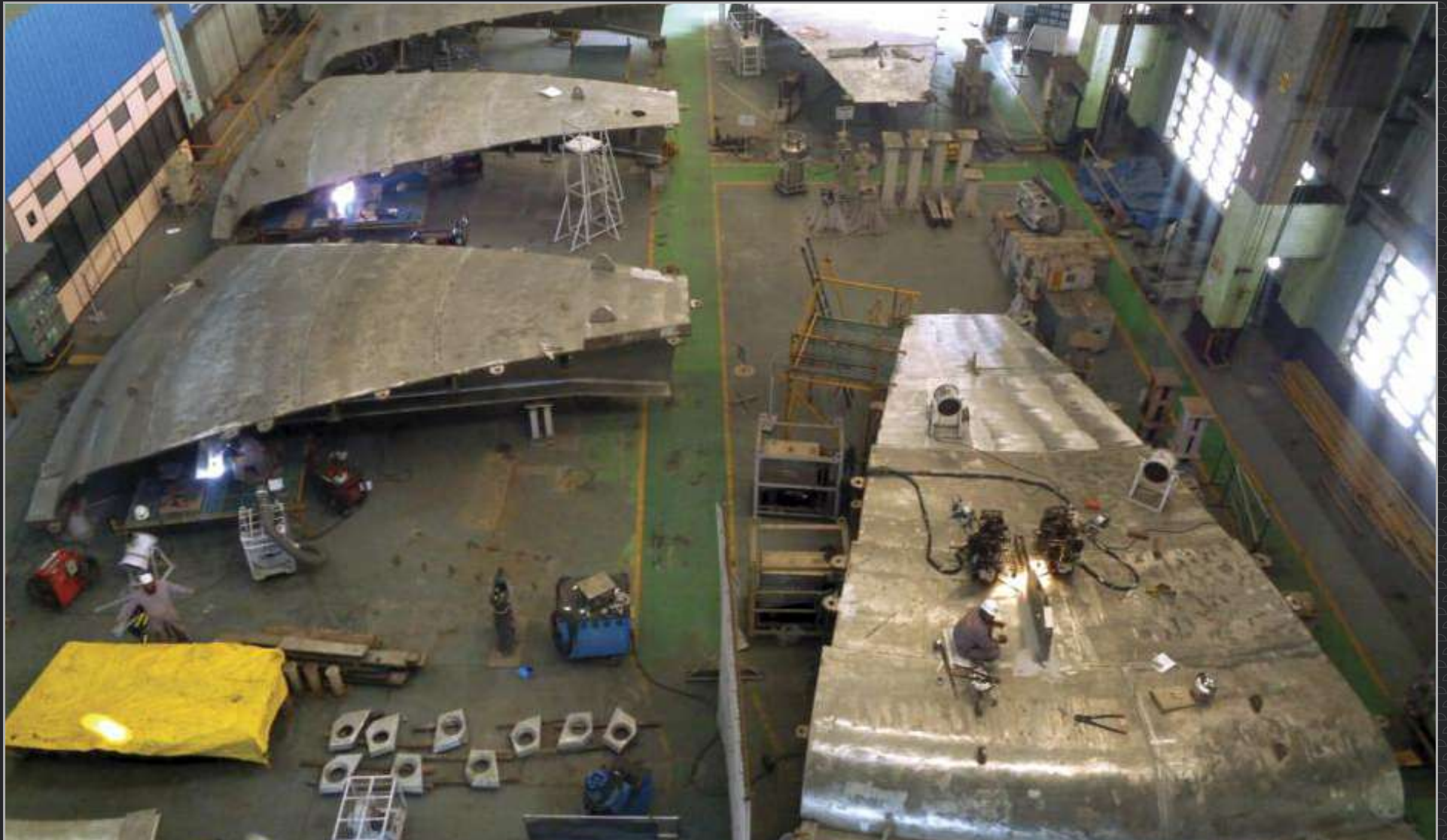
At the Larsen & Toubro factory in Hazira, India, the elements of the top lid of the cryostat are in fabrication. When completed they will be sent to the Indian Domestic Agency's assembly workshop at ITER.
