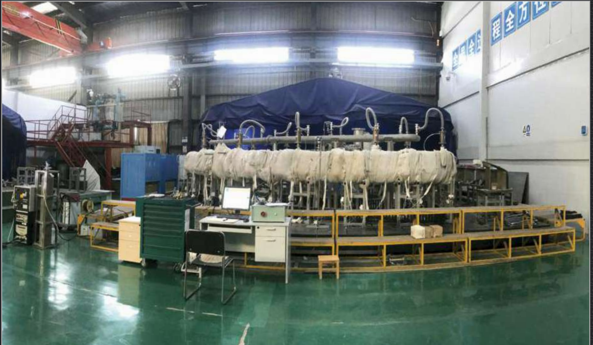
Production is underway at the Institute of Plasma Physics, Chinese Academy of Sciences (ASIPP) on the correction coils that will enable small magnetic field adjustments. Four bottom correction coils will be delivered in early 2020.
