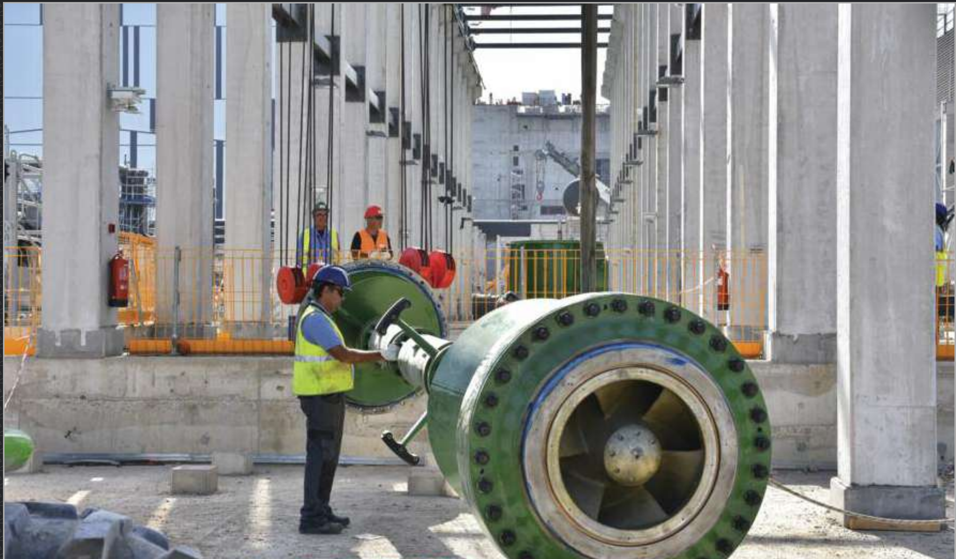
As part of the heat rejection process, 13 vertical turbine pumps will take cooling water from deep in the hot basins and circulate it to the cold basin through the heat exchangers. The six-tonne vertical shafts (pictured) must be perfectly positioned and balanced to withstand the force of the water and the rotating impellers. September 2019
