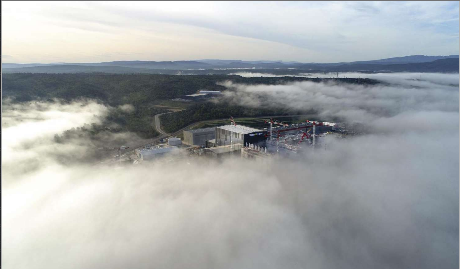
Early one autumn morning, mist from the Durance River partially obscures the construction site. ITER is nestled in the hills of Provence, about one hour north of Marseille. October 2019
