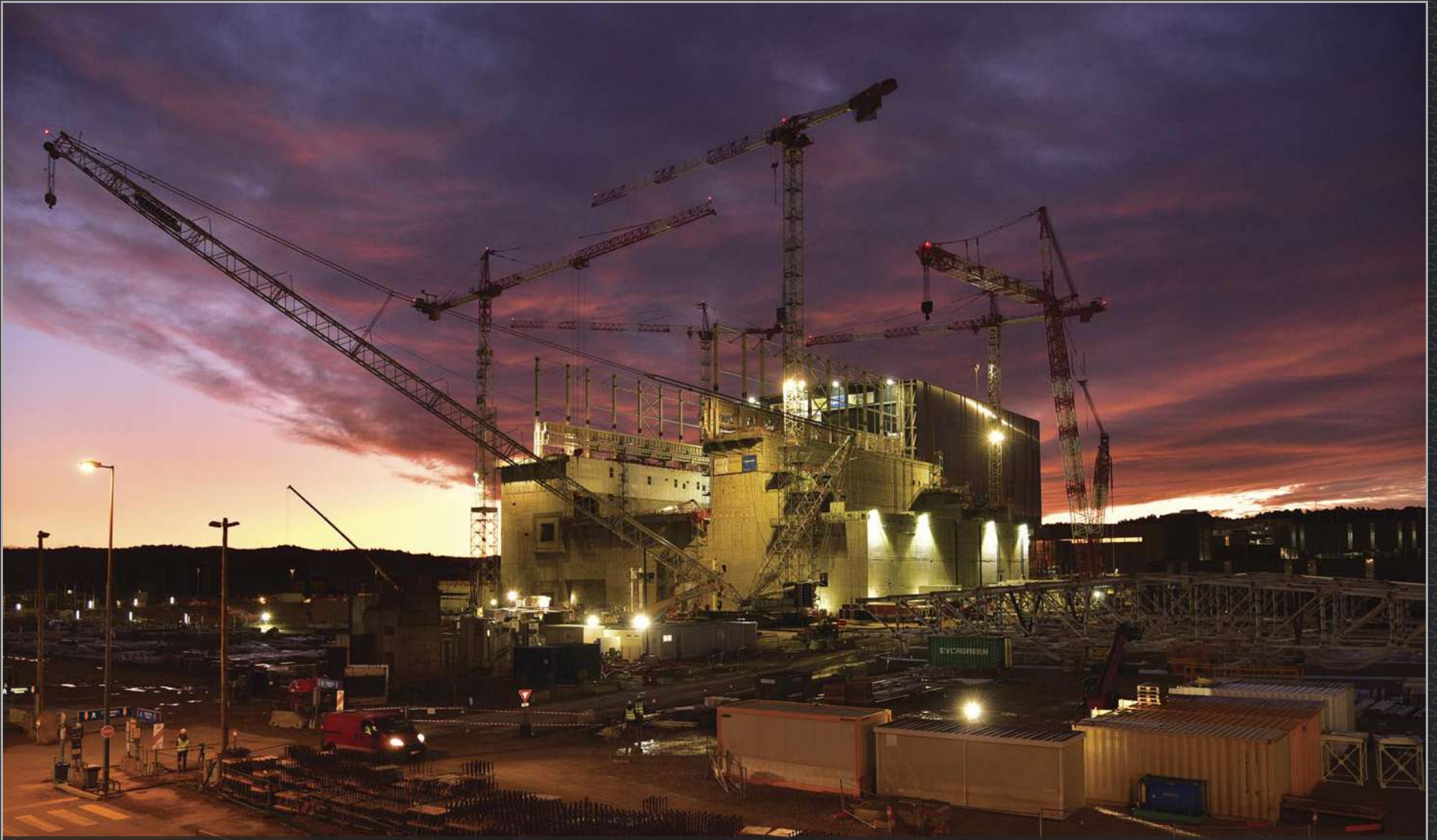
Over nine days in December, five pre-assembled modules for the roof of the crane hall are lifted into place. The first operation takes place very early in the morning. December 2019
