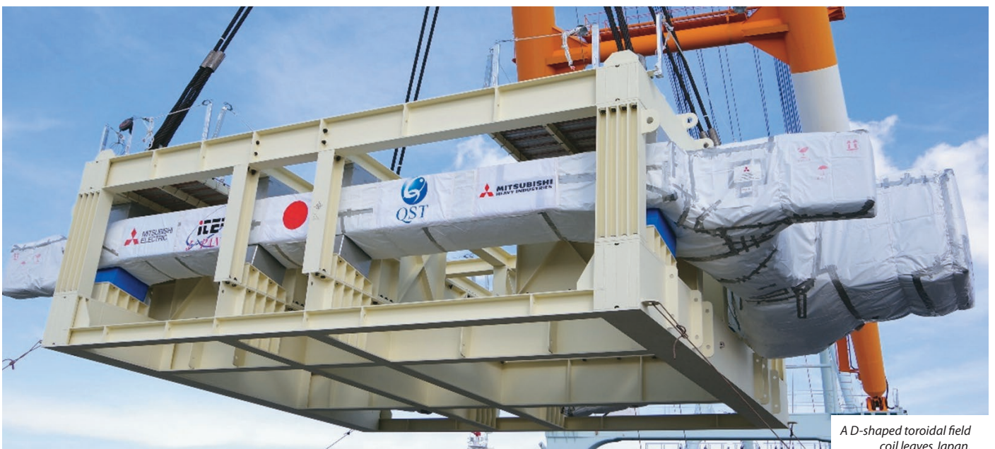
Cryoline installation in the Tokamak Complex.
