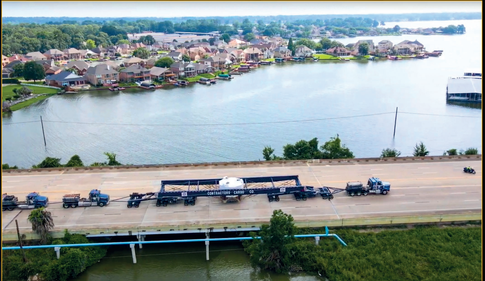
In June 2021, a massive girder truck delivers the first 110-tonne central solenoid module to the port in Houston, Texas, from its manufacturing location in southern California. A second module follows the same route in October.
