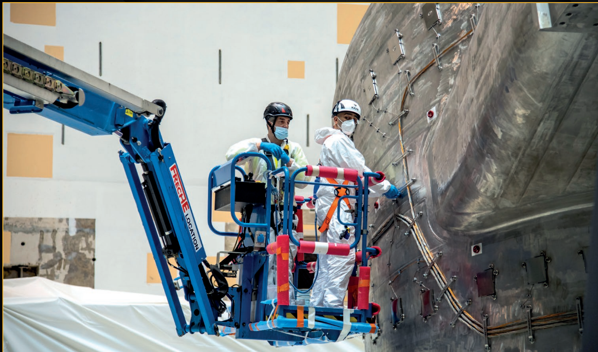
This vacuum vessel sector, still resting on its side, is being equipped with supports for instrumentation and diagnostics. March 2021
