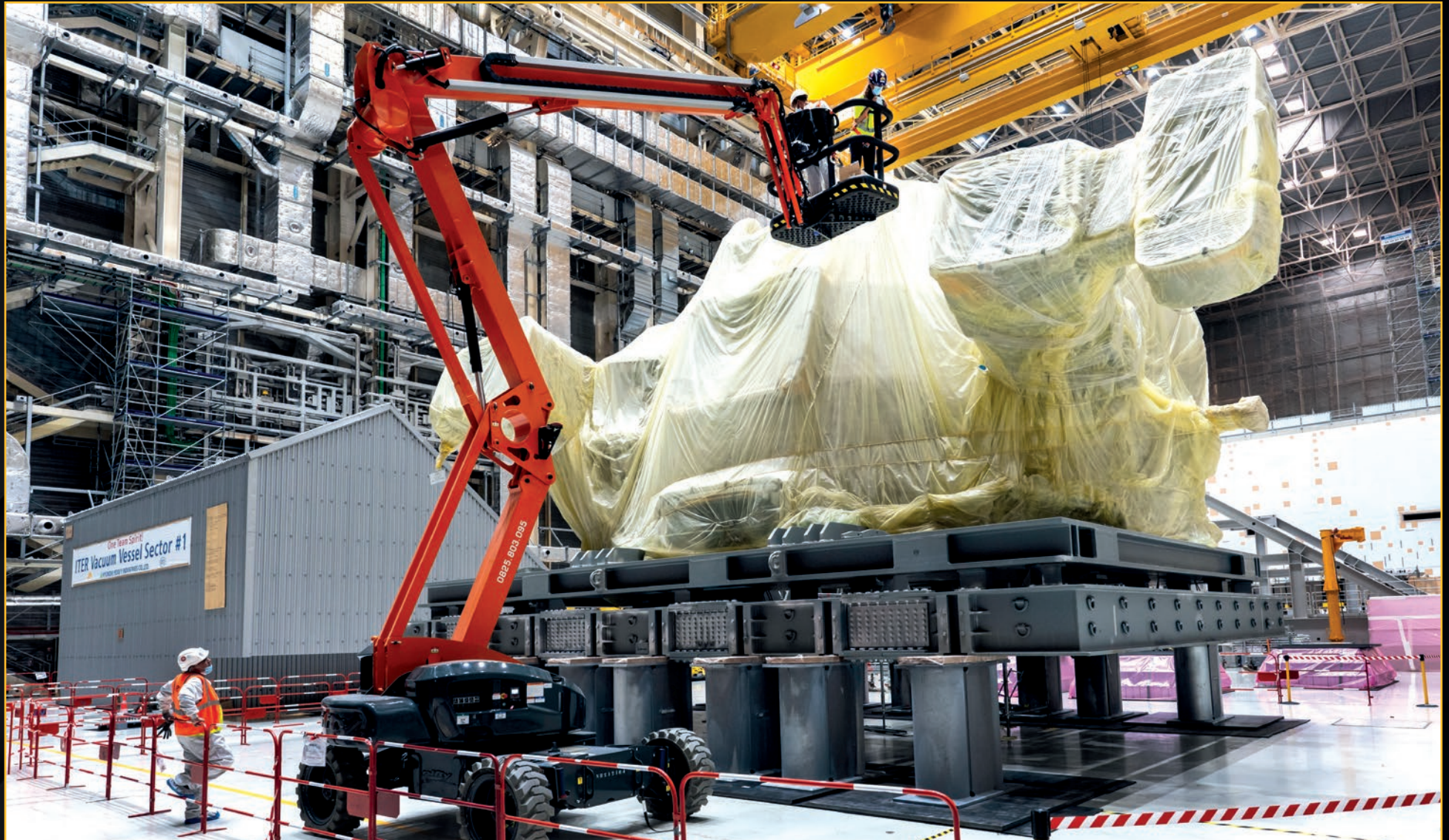
Korea delivers a second vacuum vessel sector to ITER in August 2021 (photo) and a third in April 2022. Just one sector remains to be finalized at Hyundai Heavy Industries, and it is 97% complete.
