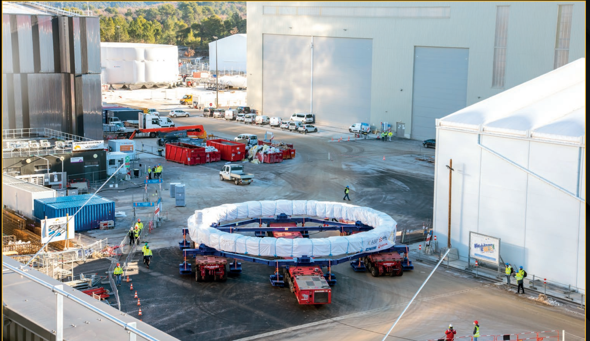
A second ring-shaped poloidal field coil (17 metres in diameter) is completed in 2021 by contractors in the European winding facility on site. Poloidal field coil #2 will be stored until it is needed in the machine assembly sequence. December 2021
