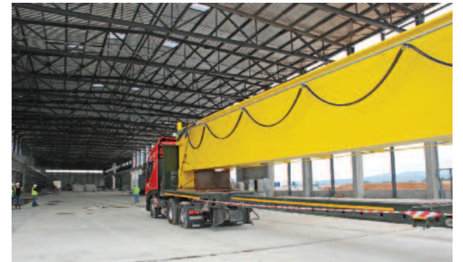
The 257-metre-long Poloidal Field Coils Winding Facility was completed in 2011.
