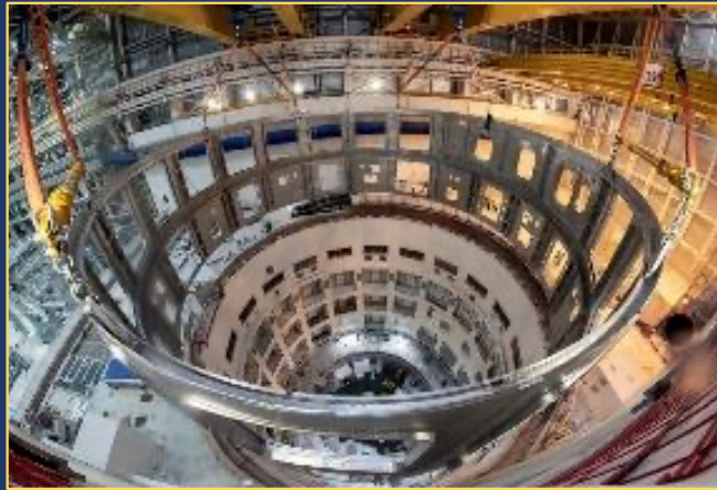
Cryostat Lower Cylinder (Aug.2020)
