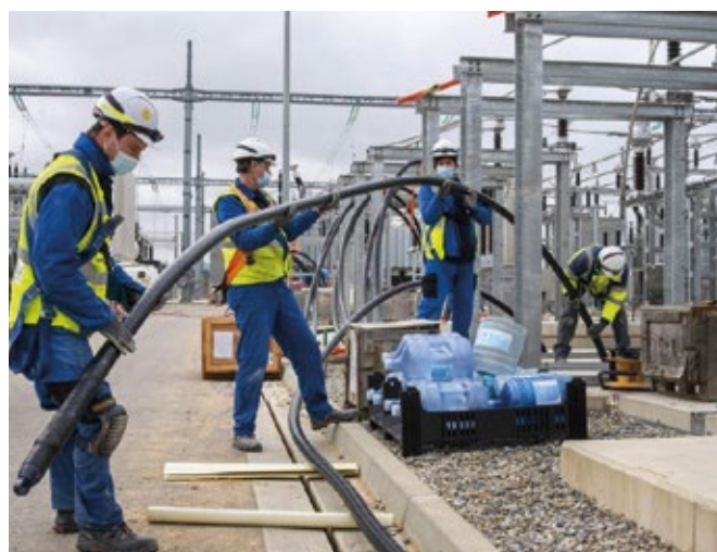
Thousands of kilometres of armoured cables run belowground in a maze of galleries to distribute power from the switchyard to the plant systems.
