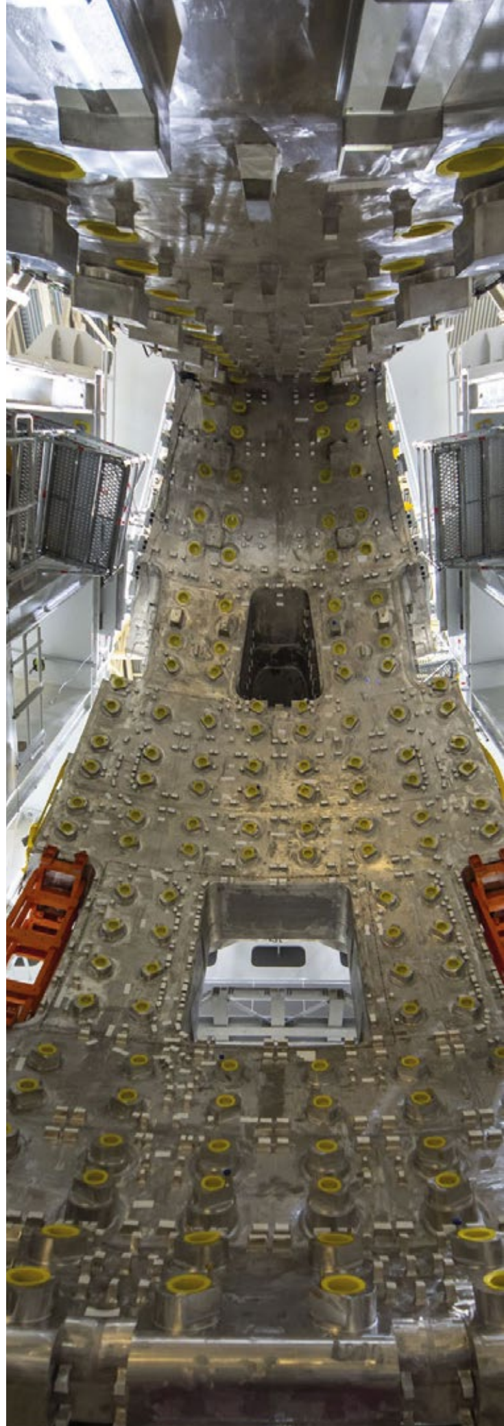
The inner surface of the vacuum vessel is pockmarked with "flexible cartridges," which are some of the interfacing components between the steel vessel and the blanket.
