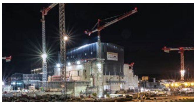
Night falls on the ITER site but work continues.
