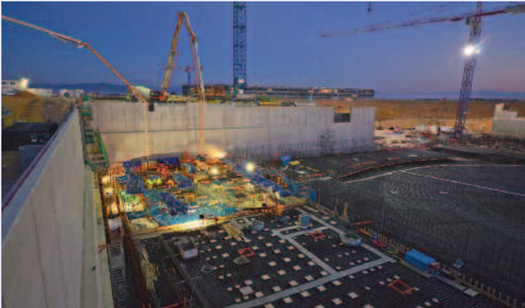
Concrete pouring for the Tokamak Complex basement begins early on 11 December.
