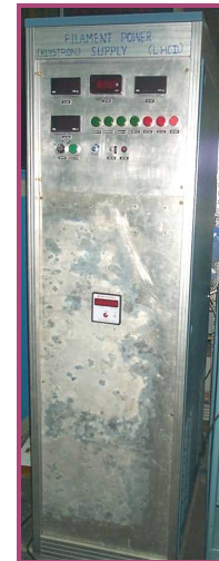
Filament PS: 12V, 50A, Soft Start 130kV DC Isolation Over Voltage & Over Current Protection.
