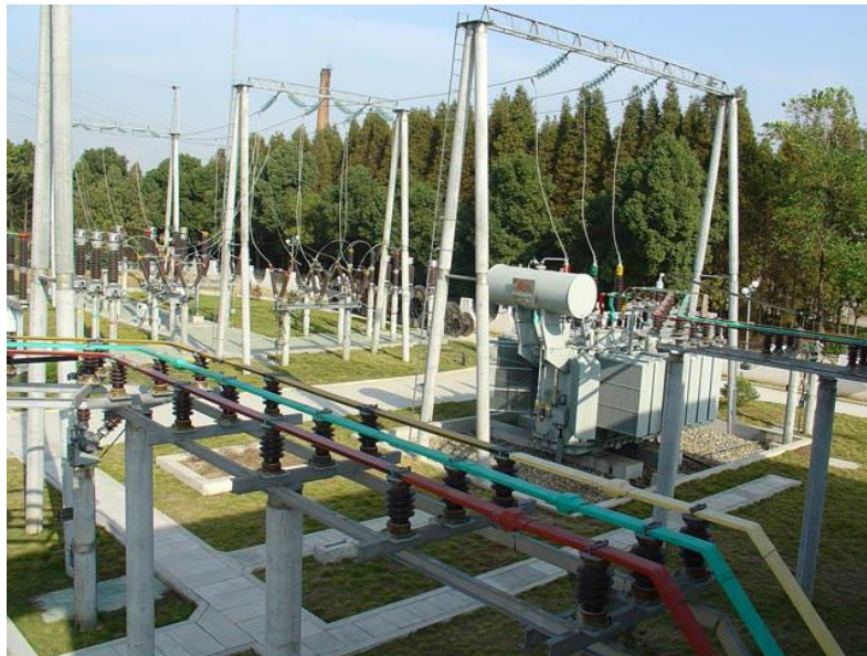
110 kV, 80 MW substation
