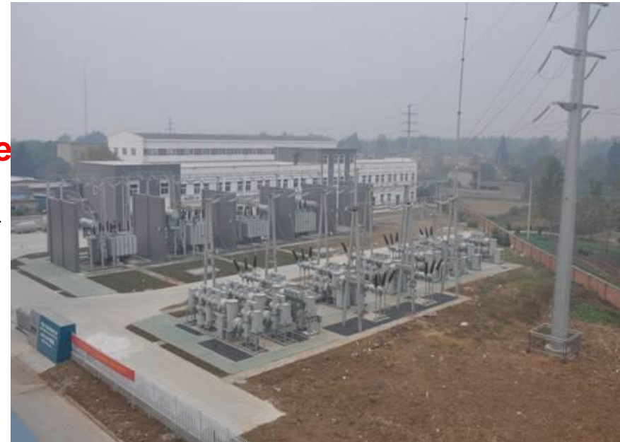
110 kV, 350 MW substation (6000m2)
